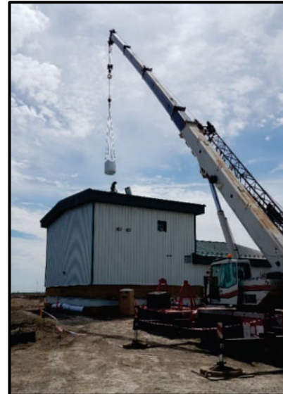
Media raised into place
