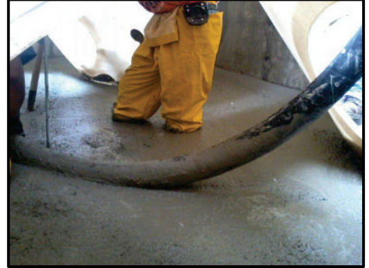
Grouting underneath multiple cones.
