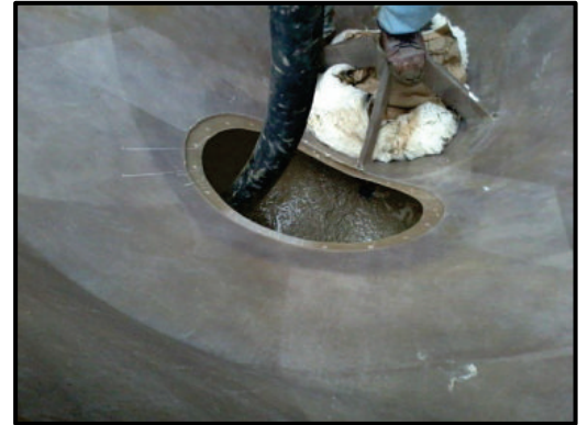
Initial grout lift utilizing the access hatch. Cup plugged to prevent spills in the bottom cup.
