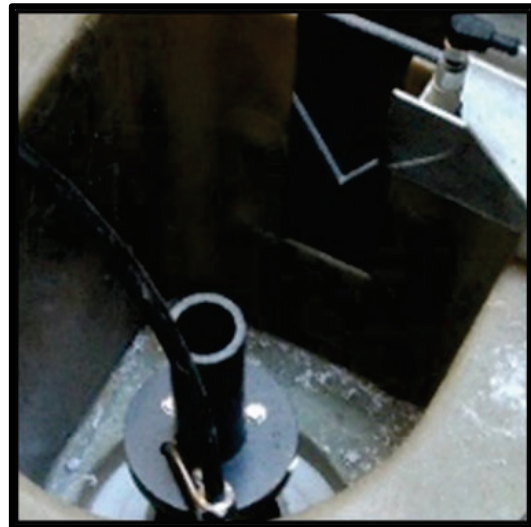
Airlift installed in washbox with temporary air supply tubing
