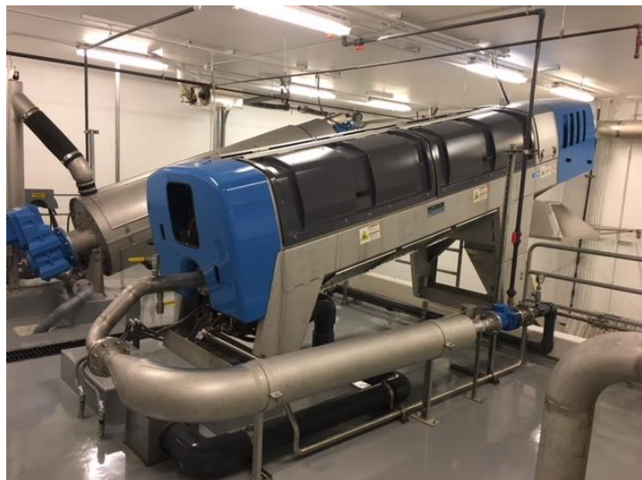
S-PRESS (background) and Q-PRESS® 620.2 Installed in Star, ID
