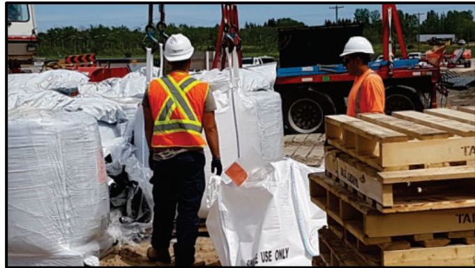
Sand Media on-site
