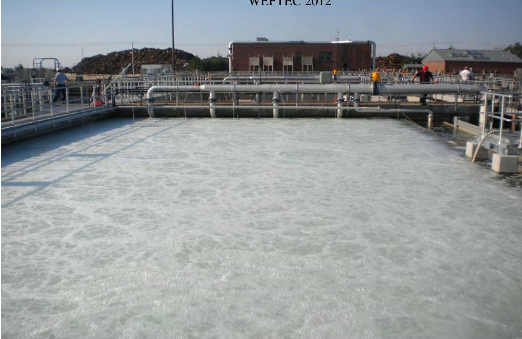
Figure 4 – IFAS Reactor in Full Scale Clean Water Oxygen Transfer Test
