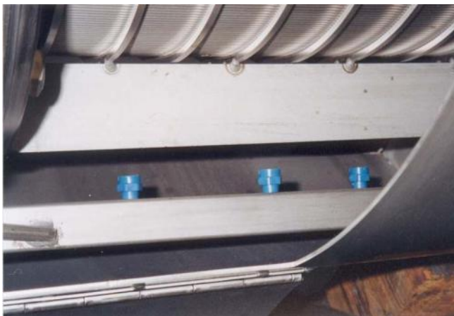
HUBER S-PRESS with High Pressure Moving Spray Bar
