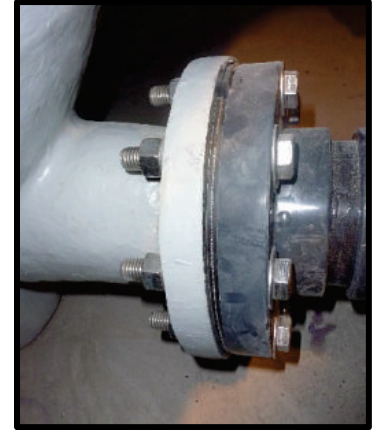
Inspection of drain screen installation with gaskets
